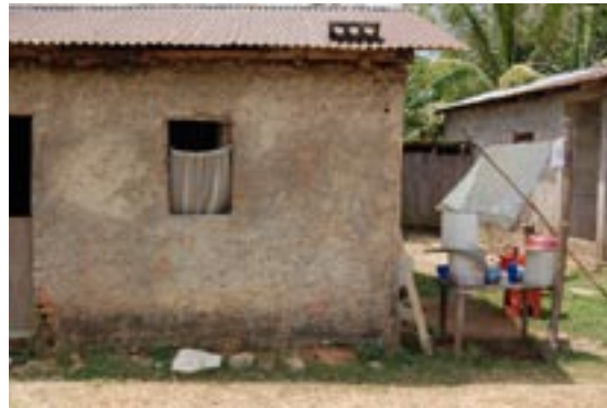
Housing is generally block wall and tin roofed, many of which are single room dwellings.
